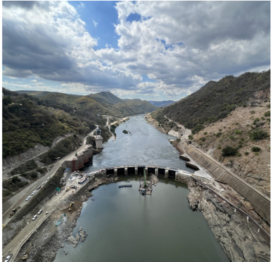
The outflow basin of the Kariba Dam leads to the Zambezi River. The small semi-circle wall was added to facilitate repairs on the plunge pool, which has eroded throughout the last 60 years and currently threatens the stability of the dam.
