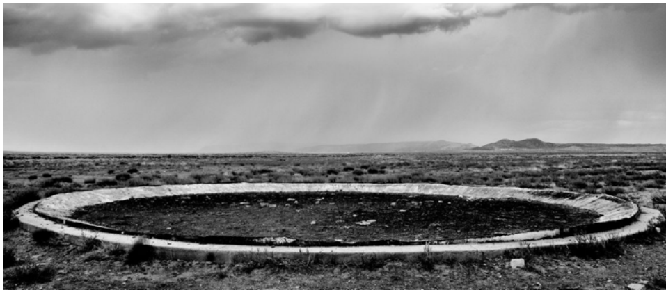
Red Mesa, Ariz. | The remains of a waterstorage tank razed because of uranium contamination; for decades during the Cold War, mines in the Navajo Nation produced the uranium used for nuclear weapons. Image by Matt Black—Magnum Photos for TIME. United States, 2019.
