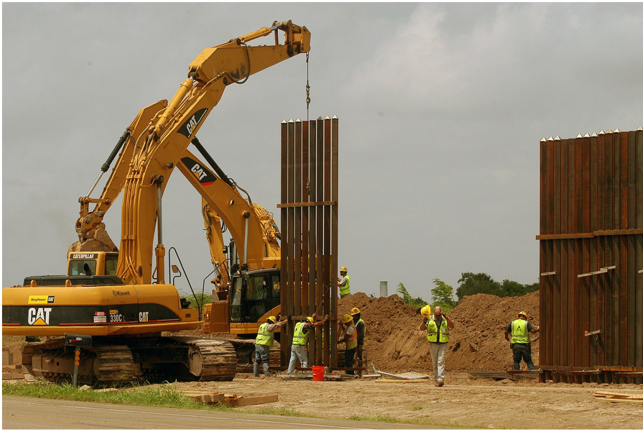
A construction crew works to erect a portion of the border fence along Oklahoma Avenue south of Brownsville on June 9, 2009. Brad Doherty for The Texas Tribune
