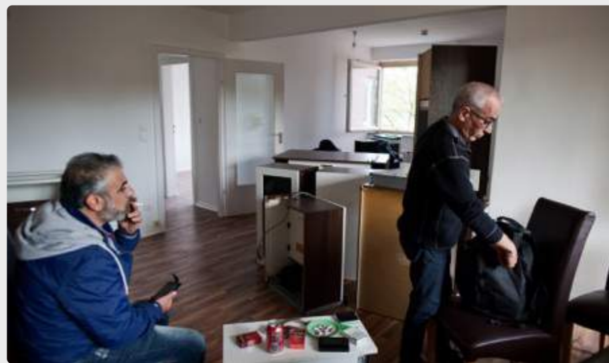
Wisam and Mwafak Al Aydi take a break from installing the kitchen cabinets and appliances in Wisam's family's new apartment in Lüneburg, Germany. The brothers were fixing up the house to prepare for the arrival of Wisam's family a few days later. Image by Holly Pickett. Germany, 2014.
